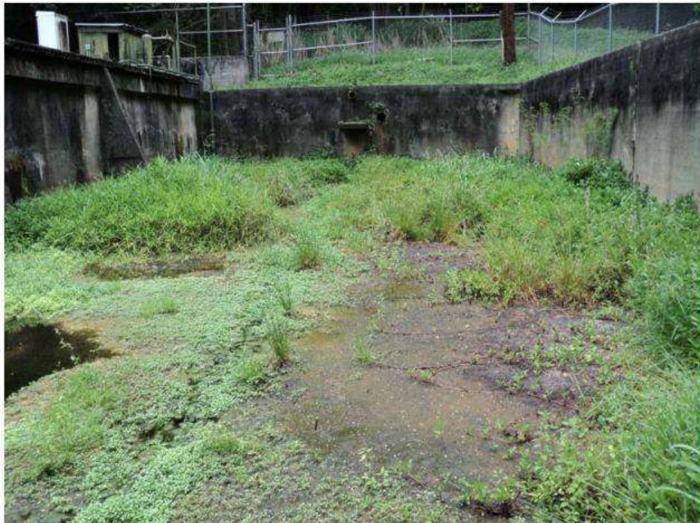
Fig. 7. Artificial Marsh at the Clearwell Parcel.
